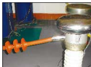
22kV 1-core outdoor termination is under testing
